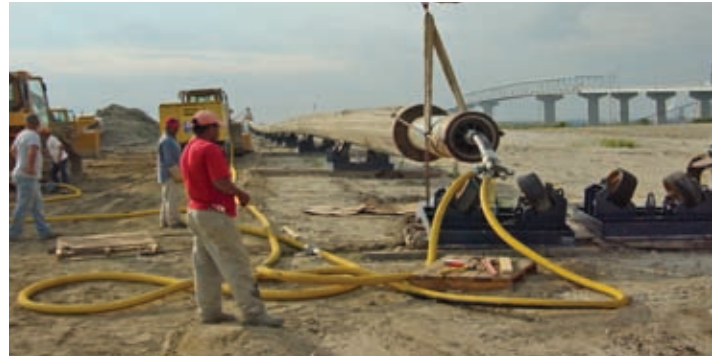
Several pipe ramming techniques have been developed over the last several years to successfully remove stuck drill stems, assist directional drill rigs during difficult pullbacks, free immobilized product pipes and even salvage failed bores by removing stuck pipe from the ground.
