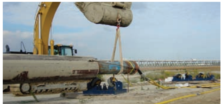
During the pullback assist the Grundoram pipe rammer is placed at the end of the pipe string. The dynamic energy of the rammer is transferred down the pipe string to the lead end of the pipe. In many cases the percussive force is enough to free the stuck pipe.
